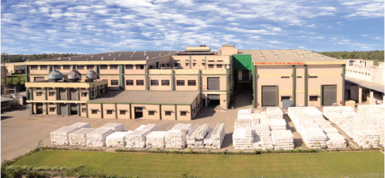
Manufacturing Plant, Roorkee
